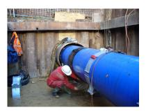
2. Wrap sleeve around the pipe joint, starting at 110'clock and passing the sleeve underneath and back over the top for the overlap.
