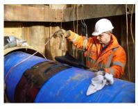
3. Heat the underside of the closure strip with 4 passes of the propane torch and place over the overlap. Install the closure strip properly before heating the rest of the sleeve.
