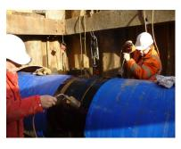
**5.** Check edges of sleeve to ensure mastic "wetting out". Use a roller if needed.
