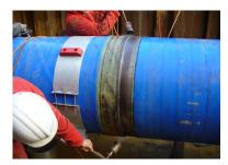
I. Clean joint with power wire brush to ST3 minimum & lightly abrade adjacent coating. Degrease using cleaner and clean rags. Preheat pipe to 70°C (temp. sticks will be provided).
