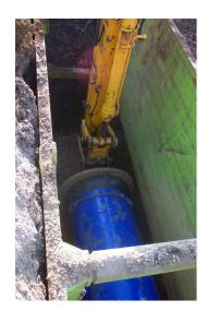
Where suitable equipment is available on site, push fit type joints can be made using a trench digger. This method reduces the time required to make a joint.
